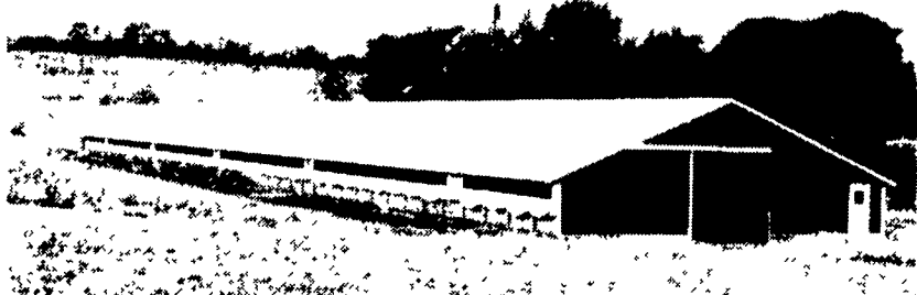
50'x520' Starter & Grower Turkey Building, Starter Building With Wood Trusses, Tri Ply Ceiling, Insulated Sidewalls.
