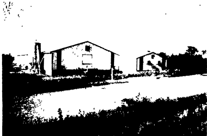
High Rise Building w/Egg & Cooler Room, Partial Block Walls, 2x4 Framing, Steel Siding, Aluminum Roofing & Certified Trusses
