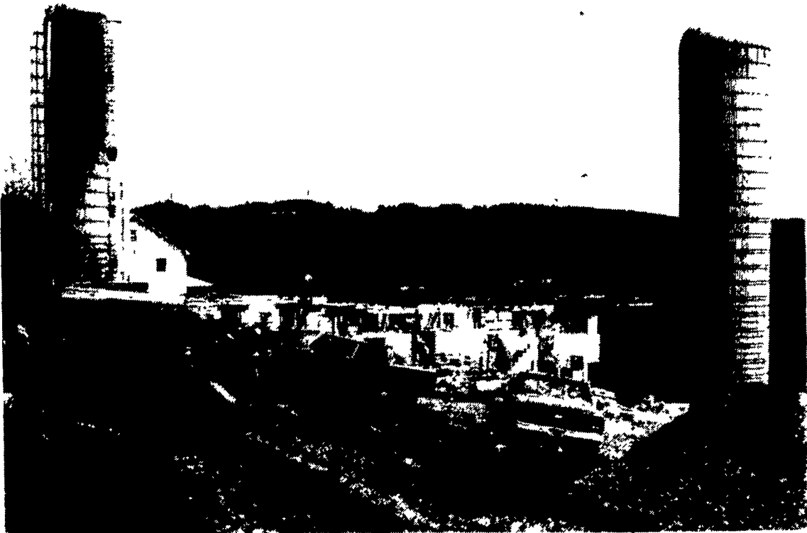
Rebuilding was well underway Thursday of the John Esch barn destroyed by fire Tuesday afternoon. Damages were estimated near $100,000 at the farm in New Providence.
