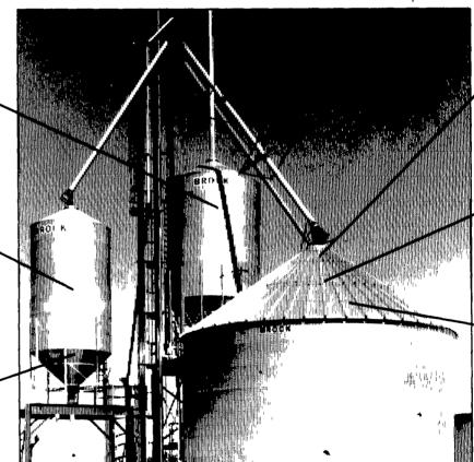
High rise (3" high) roof ribs provide tight fit & added roof strength
