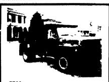
F700---24 500 GVW 370 V8 5 Speed 2 Speed Rear Tilting Hood PS Perfection Dump Body
