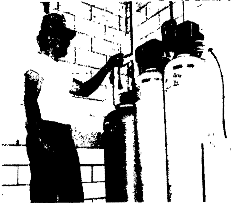
Strasburg dairyman John Good adjusts the valves on his sulfate tank. Two taller tanks in the foreground remove nitrates.
