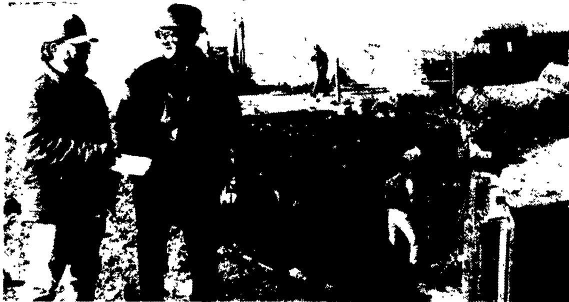
David Pierce, on left, describes to Charles Harris, Cochranville, chairman of the Chester County Conservation District, the operation of his manure handling facility.
