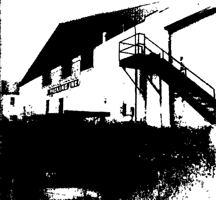
Weeds crowd the outside yard, but there's still enough potential inside the Clover Meat Packing plant to make a co-op takeover worthwhile, organizers believe
