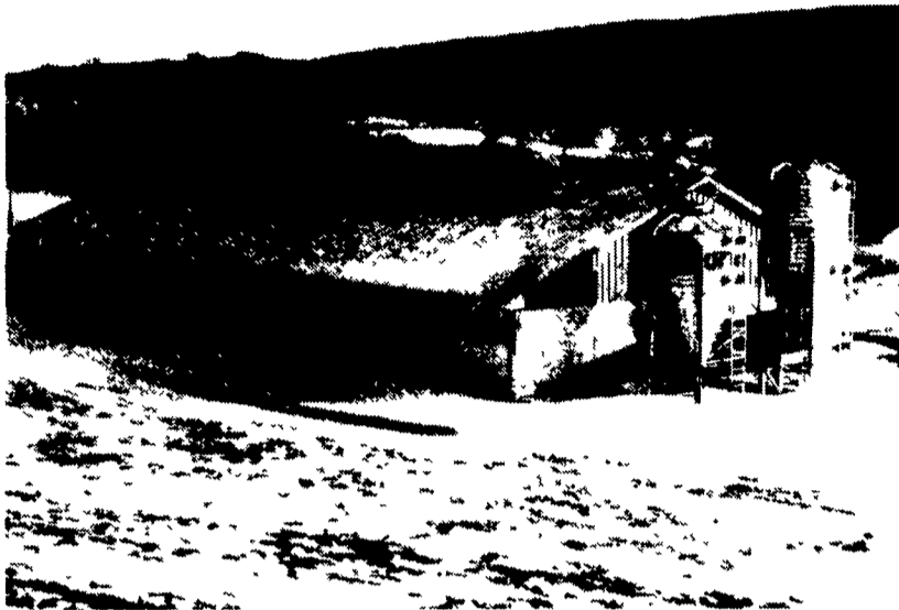
Natural Ventilated Unit
