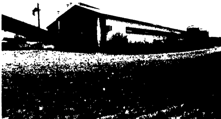
Uniarch Natural Ventilation Barn With Curtain Southside, Insulated Vent Doors On Northside And Adjustable Ridge Vent At Peak
