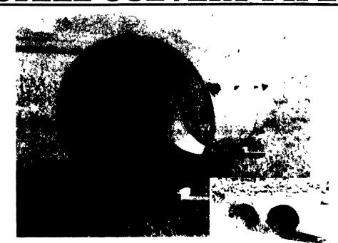
Used carbon steel storage tanks which we have removed the end (heads). Lifting lugs attached. No coating. These tank shells make an inexpensive, quick and strong bridge. Tank shells burjed with 3 feed of ground cover can support 80,000 lbs.
