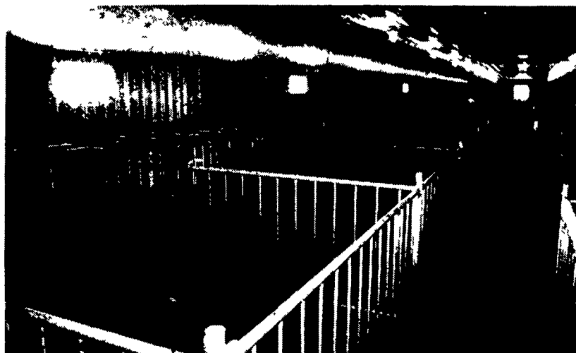
Hot Dipped Galvanized Breeding Pens Over Concrete Slats.
