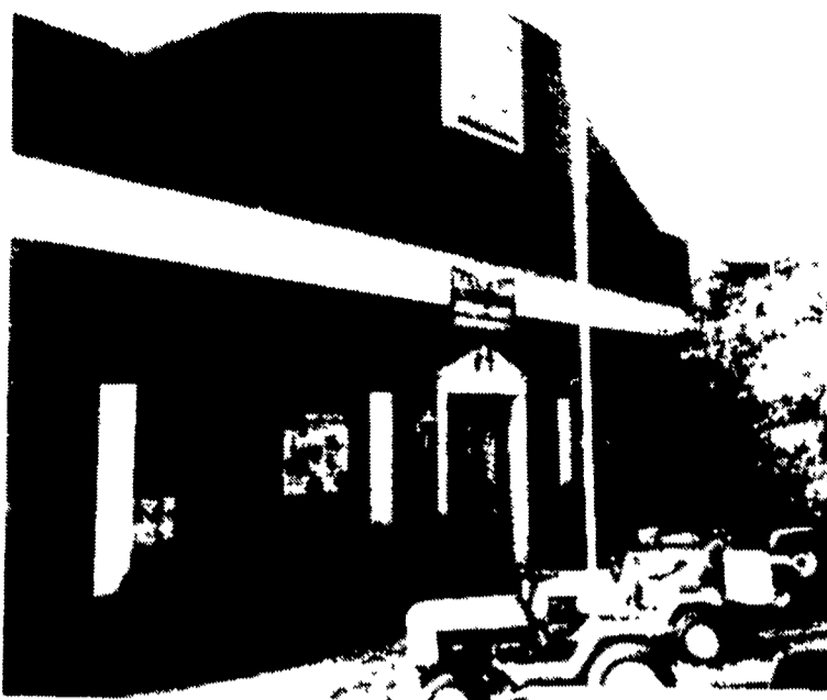
Trenton Ford Tractor, Inc. at 2836 Brunswick Pike, Trenton, N.J. has its ultra-modern facility on 3.5 acres of ground.
