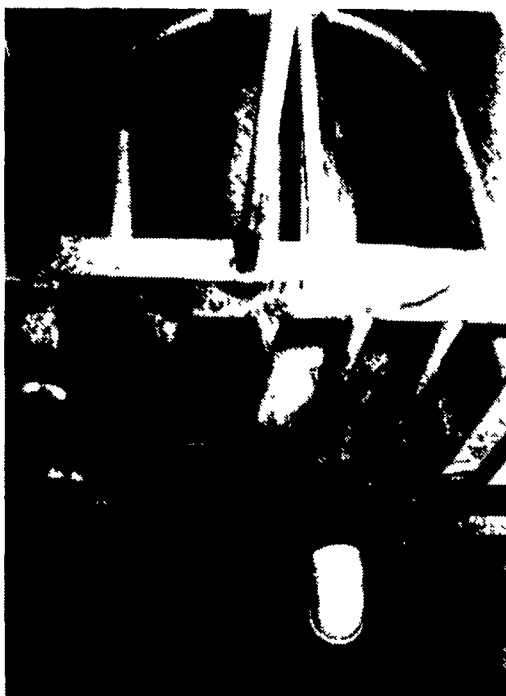
6. Cooling is provided through snout pipes located at head end of each farrowing crate. Pipes are linked underground to geothermal tubes.
