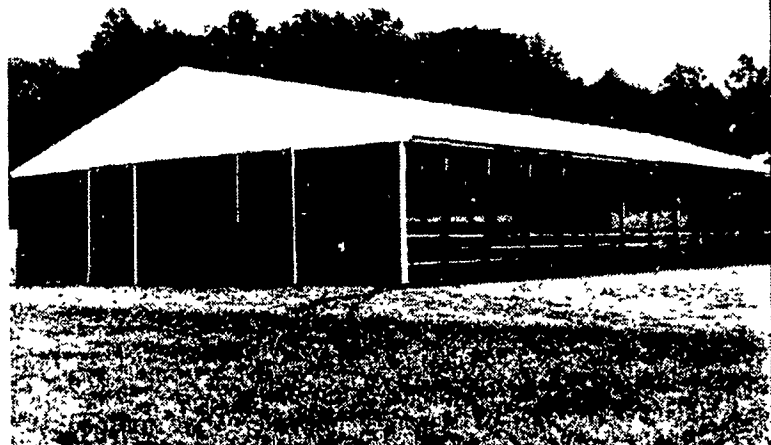
This 60x120-foot indoor arena was completed this summer by Ned and Donna Bean, and will allow Donna to continue to train horses and give lessons throughout the winter. It will eventually have stalls and a washroom added to both sides of the building to accommodate what Donna hopes will be an expanding business.
