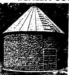
Did You Know Behlen Corn Cribs are No. 4 gauge, which is heavier than most other brands and helps to prevent bulging of sides.
