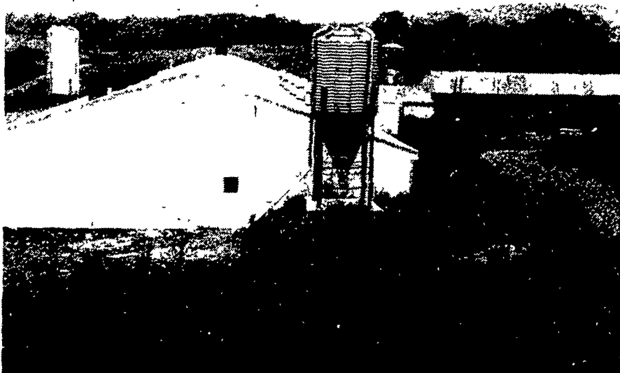
All New 250 Sow Gestation, Farrowing And Nursery Building
