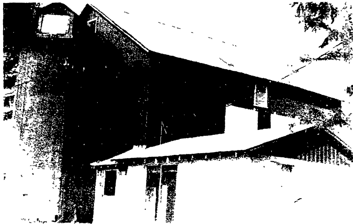
New milk house has been added to front of barn. Wood silo will become the barn office and will feature hexagonal windows.
