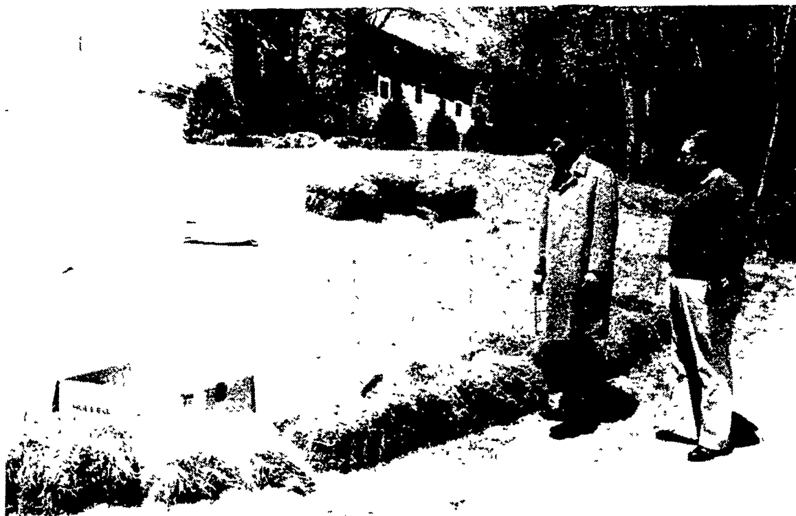
Bales of hay, when properly installed, can protect neighboring property. Richard Laudenslager, left, Soil Scientist, Department of Environmental Resources and Ted Kaufman, Project Engineer for Great Valley Corporate Center, Malvern, compare notes on the proper installation of hay bale sediment control.
