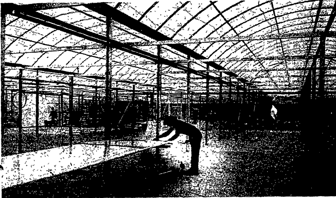
A worker cuts plastic panels that will form the walls of the Pepperidge Farm greenhouse, which is now being built near Pennsylvania
