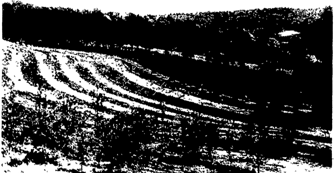
Contour strips are still used on Bear Mountain Orchards steep hillside to control erosion. Diversion ditches also were added to the orchard — some of the longest ditches in the county.
