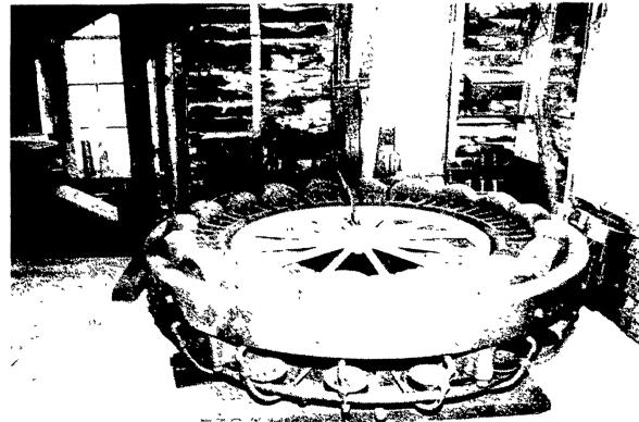
With the addition of the West tire shrinker. the wagon works switched from hot to cold ironing of the wheel tires. Before, the iron tires
