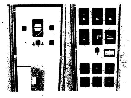
This switchgear enables you to sell power to the power company automatically, when you have surplus, and automatically draw from the power company when you need it.
