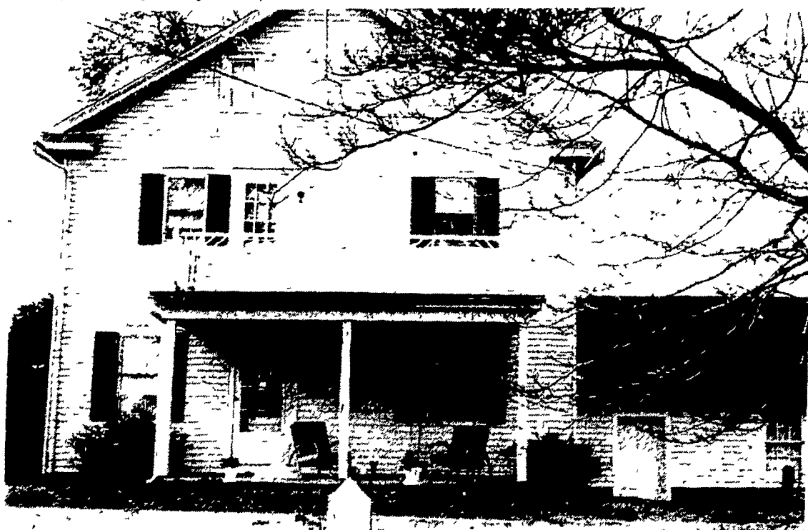
This three-story house was attached to the original farmhouse but in 1883 it was hoisted from its foundation and moved several yards via logs and a team of horses.
