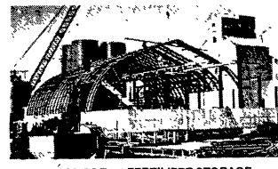
66x80 Foot FERTILIZER STORAGE 2,600 Ton Capacity South Dakota 50' - 100' wide to meet various requirements & capacities
