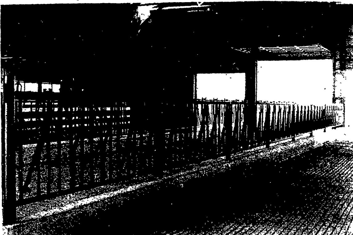
The new freestall barn is equipped with all the latest equipment, including the head-lock partitions for quick-catches of cattle.
