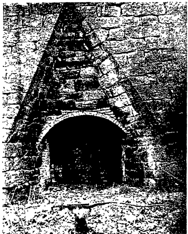
Forming a geometric marvel of perfectly placed stone, this entrance to the furnace stack in the casting house formerly spewed out molten iron every 12 hours. It flowed across a sand floor to pig molds, there it was cast into cannon balls, stove plates, etc.
