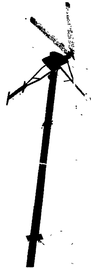
This windmill was one of the featured exhibits at the J&J Agri-Spon Products Energy Day held last week. The windmill is used to preheat the water that heats the Agri-Spon building, site of the field day.
