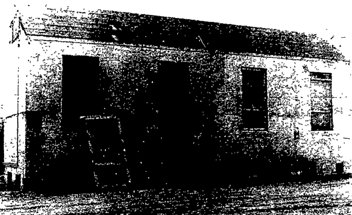
Hay bales and other potential commodities can be stacked for solar drying in four separate chambers, 11 feet square by 14 feet deep. Wilmot's homemade monometer, (looks like a
