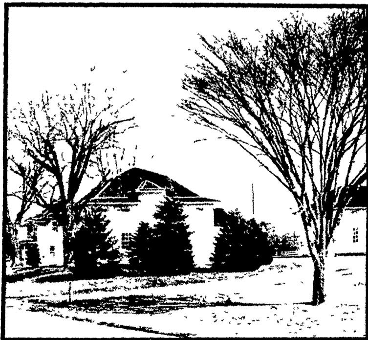
This Milton Hershey barn is disguised under a unique roof — four sides angle up at three levels before meeting at a center peak. This style roof matches the one on the adjacent house and smaller shed.
