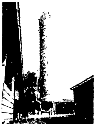
THE TERRE HILL CONCRETE STAVE HERD BUILDER BOTTOM UNLOADING SILO
