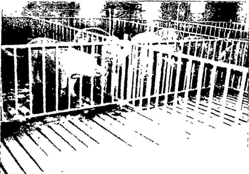
GESTATION & BREEDING ROOM WITH HOT DIPPED GALVANIZED SURE-LOCK FENCING & CONCRETE SLATS.
