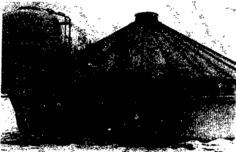
Wilson Rohrbach, right, and son Roy of Mertztown, Berks County have constructed the first round finishing barn for hogs of its type in Pennsylvania. The fully-insulated metal building uses a conventionally-sized grain bin roof for its design and construction.
