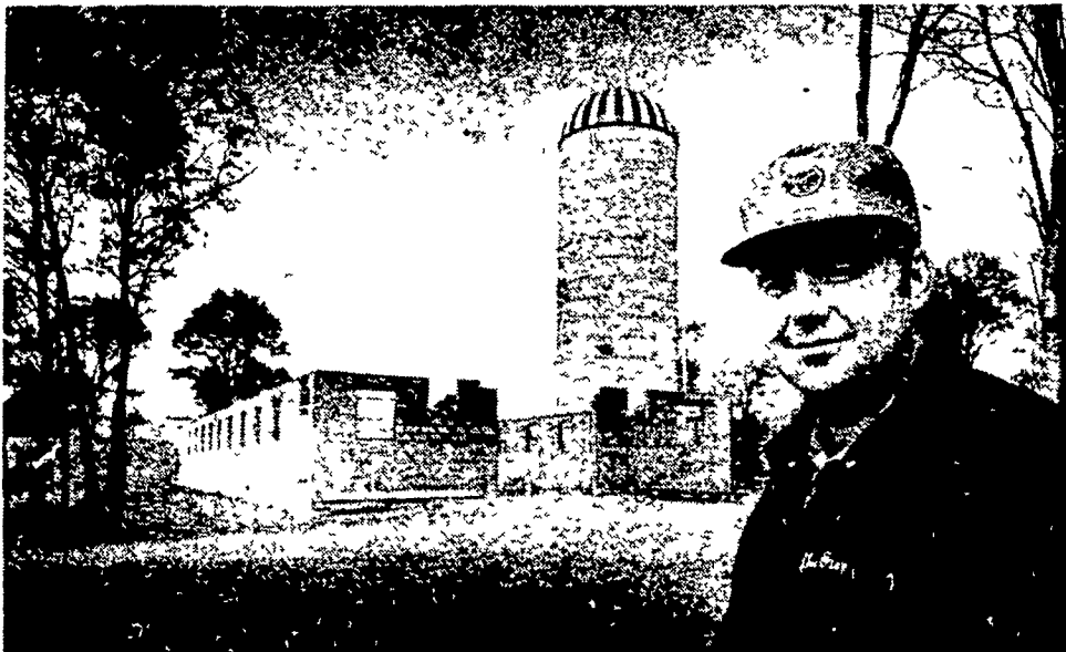
Dairy training center under construction is shown with Robert Barr, president of Walk-Way Vocational and Bible Institute.
