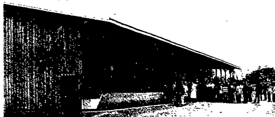
Robert Heffner's feedlots, located near Fleetwood, Berks County, showed the beef producers a new face to a metal pole building. Heffner tacked wooden siding on his barn to keep the cold winter air out like snowfence traps snow.
