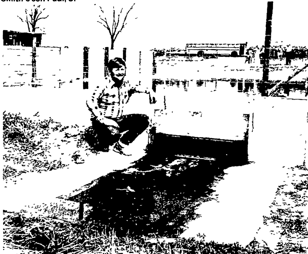
J. Parker Smith poses near the liquid release board of his new solids separation pit. Parker was the first farmer in the nation to complete a pollution control structure under the new experimental Rural Clean Water Program.
