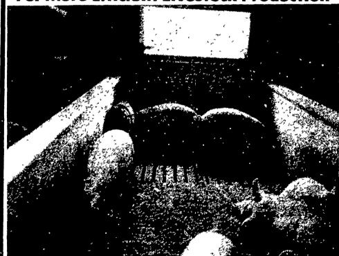
These steel reinforced concrete slats are available in lengths up to 10 feet in the gang style, and 12 feet in the self-spacing, individual style.
