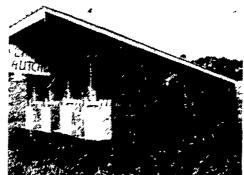
Room for 4 calves, overall size 8x12 with 3' overhang to protect feeder on 4x4 treated skids, moveable, 1/2" plywood sides with white baked enamel roof
