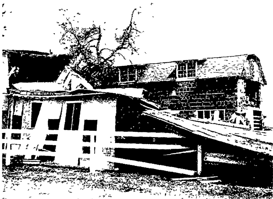
This 75x40 barn on the Clyde Deck dairy farm, Ramona Road, Jackson Twp., lies broken by the storm. Note blown-out wall on barn in background.
