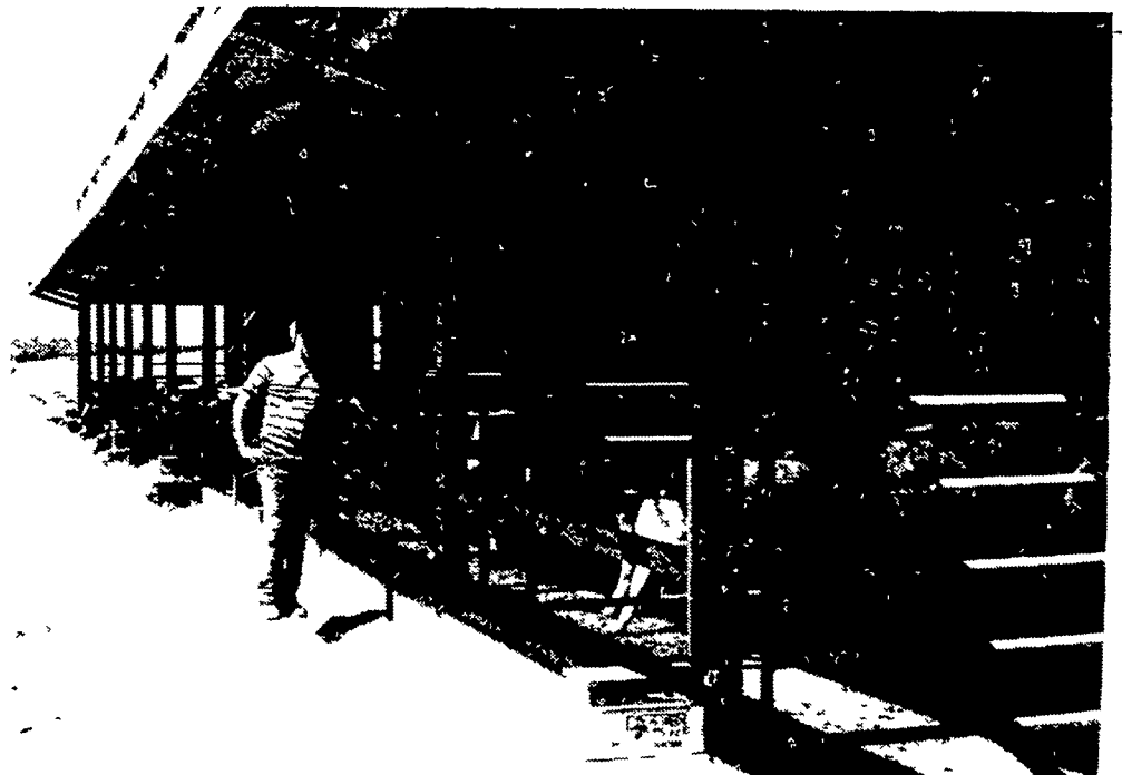
Roof-covered feeding area is pointed out by Abram Barley, Jr. Adjustable head-locks will be installed later to replace the temporary plank enclosure.
