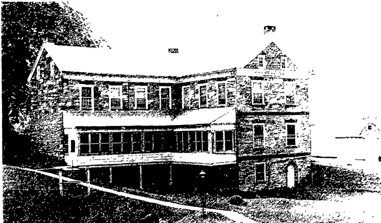
Large stone home, called the mansion or plantation house in old records, is found on the dairy farm of Arthur and Liz Schlappich, northwest of Leesport. Exterior features include red sand-
