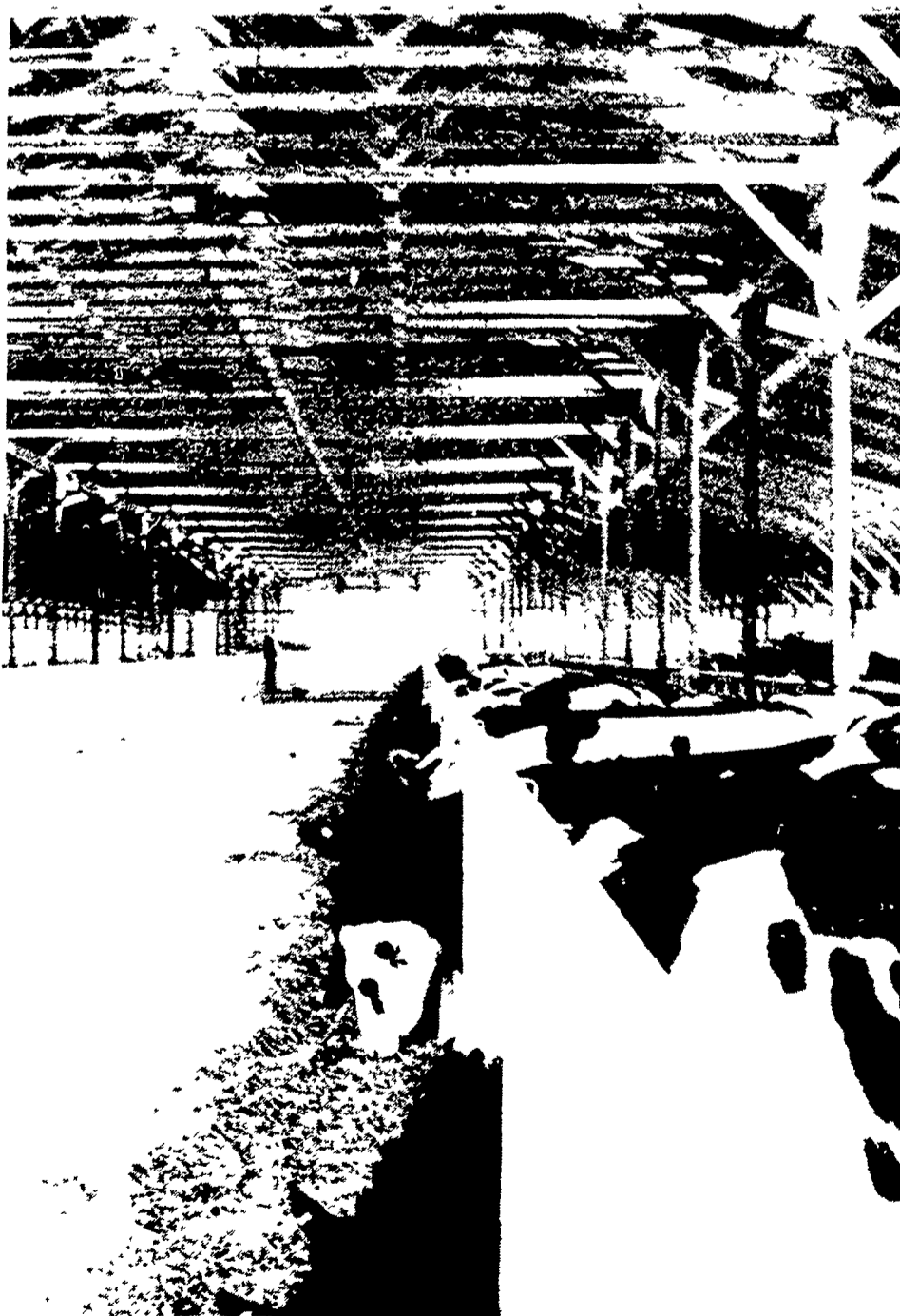
Wide central aisle will permit more efficient drive-through feeding with a mixer-wagon in the 412-foot-long barn at Oregon Dairy Farm.
