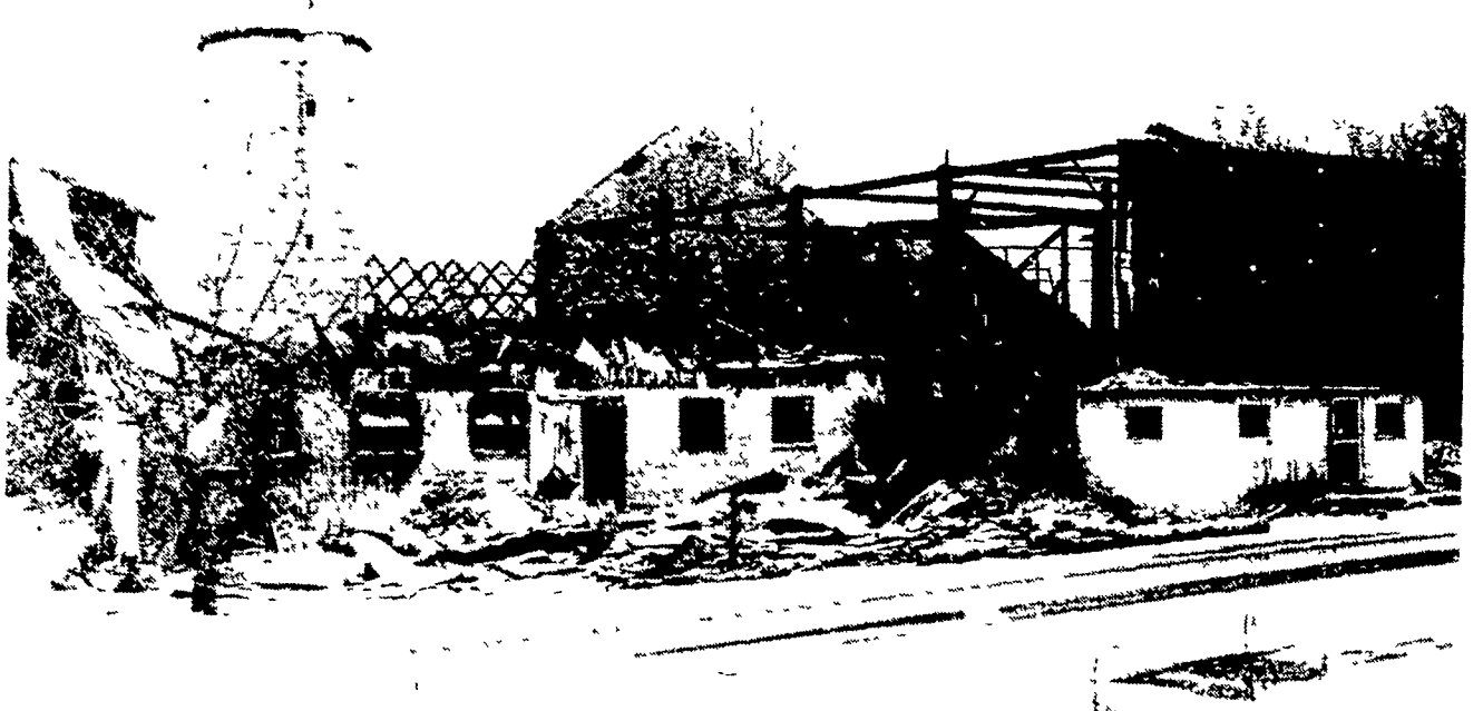
Concrete silo, stone walls and smoldering skeleton are all that remain of a large barn
