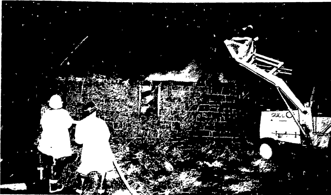
Firemen in a bucket loader shoot water over the remains of the Philip Seppi barn in Brickerville. High winds fanned the blaze and sent billowing
