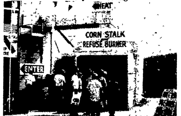
Front view showing the large, wide doors where the bale is put in.
