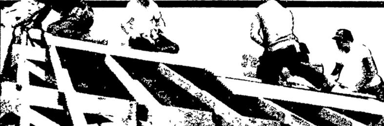
Onduline sheets are the perfect combination of strength and durability, yet they're lightweight and easy to handle. Even farmers with no roofing experience can install Onduline themselves, using either nails or screw fasteners. All you need is a saw and hammer or power screwdriver
