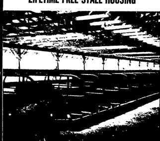
Cut bedding costs 75 per cent, reduce labor for barn cleaning and cow washing, reduce teat and udder injury to the minimum — house your milking herd in free stall housing. Each cow provided a stall for loafing. She won't be stepped on, the rear curb forces manure out into alley for mechanical cleaning or washing. A few minutes twice a day cleans the stalls and curbs, bedding lasts almost forever if your stalls fit the cows Popular sizes are 6'6", 7' and 7'6" Size 'em by breed.
