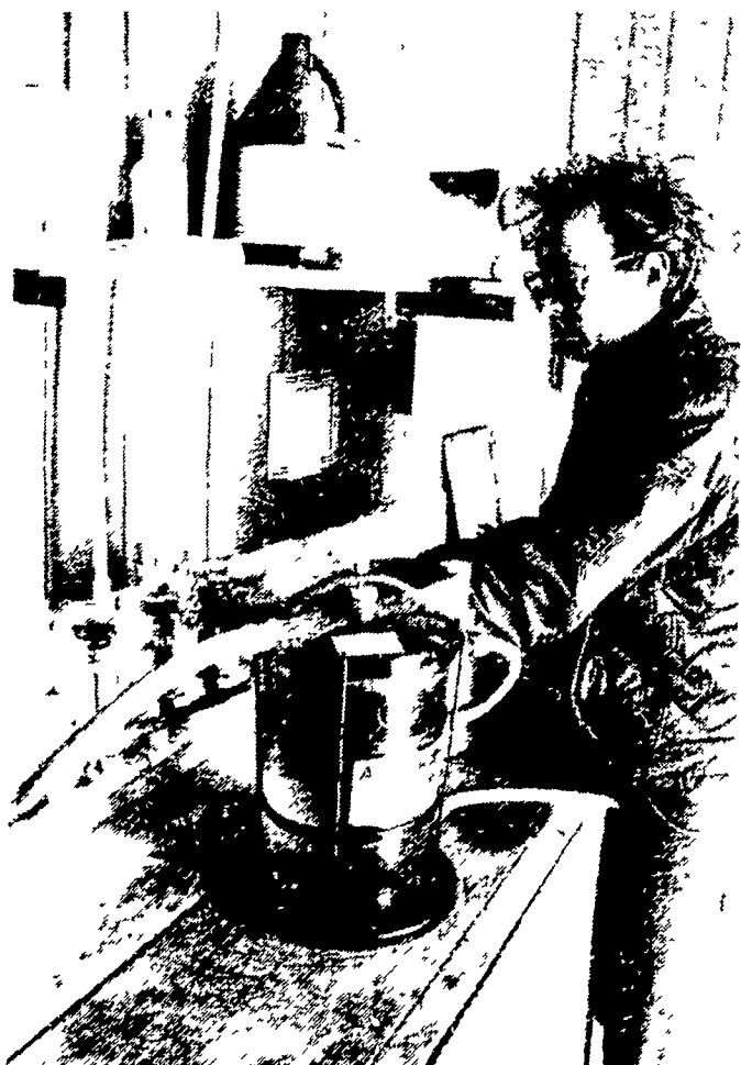
Joe Zimmerman used this metering device in the service room to medicate portions of his watering system. Medicated drinking water can be directed to any one of four housing sections.
