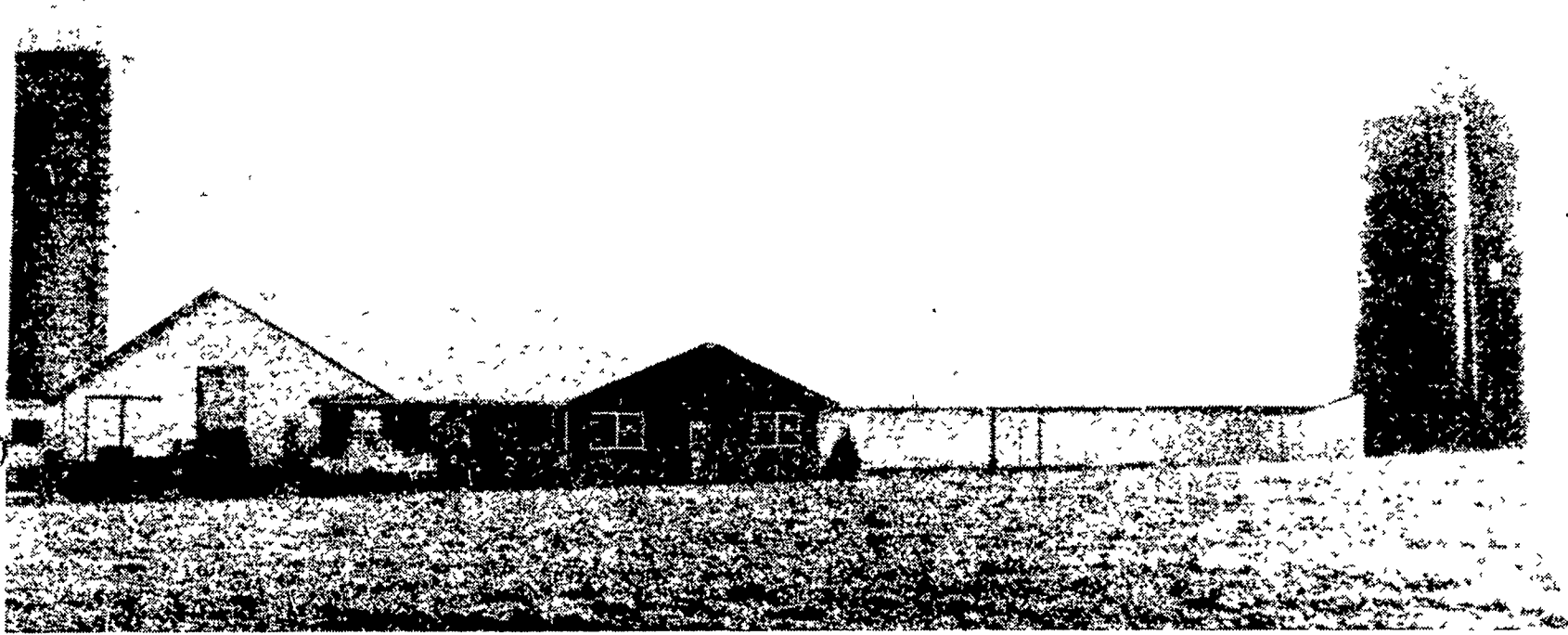
This is the newly built dairy barn at the John L. Landis farm which was open to inspection last weekend.
