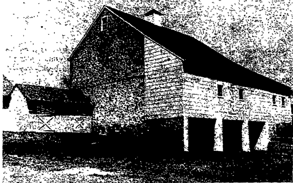
This great stone barn has been preserved and refurbished. The sleek, white conical supports under the forebay are typical of the ap-
